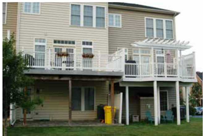
RECOMMENDED - Townhouse decks with traditional vinyl picket rails, trellis and orderly under deck storage.
