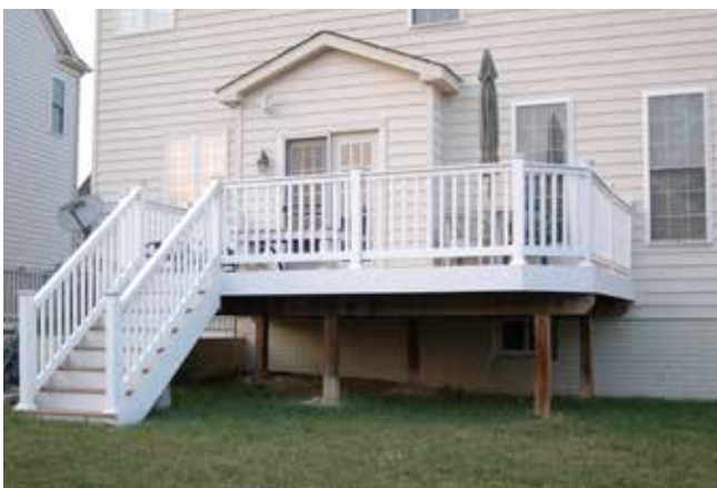
RECOMMENDED - Single family properly scaled raised deck with vinyl stair and rails matches the house color.
