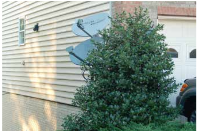
RECOMMENDED - Ground-Mount Satellite Dishes are concealed behind landscape and shrubbery screening.
