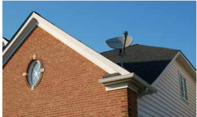
RECOMMENDED - Roof-Mount Satellite Dishes are concealed behind roof structure at rear side of homes.
