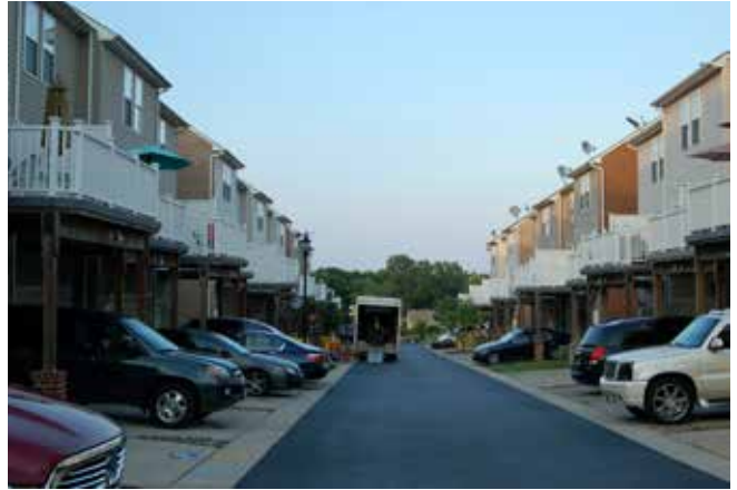
Rear Alley facades
