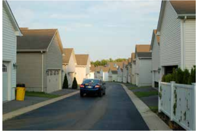
Rear Alley garage facades
